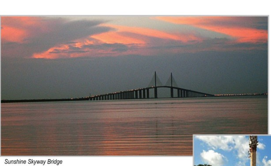
Sunshine Skyway Bridge
